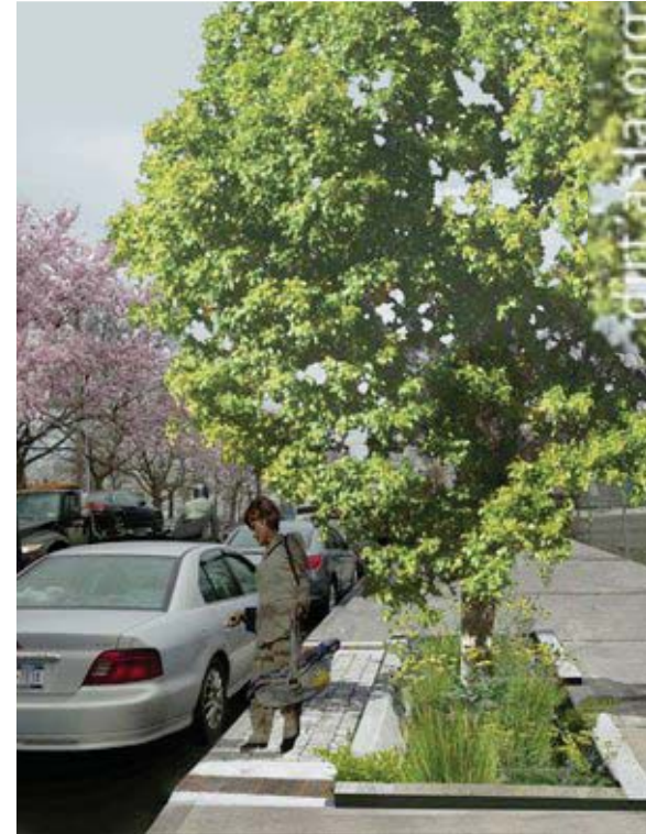
Curb inlets, permeable pavers, and tree filter box
